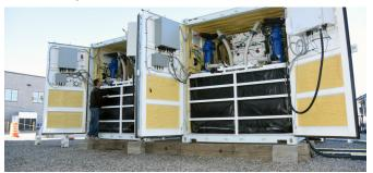
Figure 5. Flow battery at Idaho National Laboratory's Microgrid test bed. Source: U.S. Department of Energy
